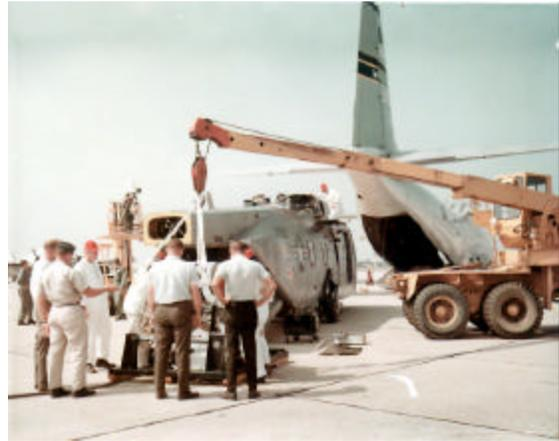
We can now pull the helicopter safely into the C-133. All loading was done with the C-133 loadmaster supervising. With one CH-3 fuselage in place next came the two transmissions on their stands and the two APU storage boxes.
