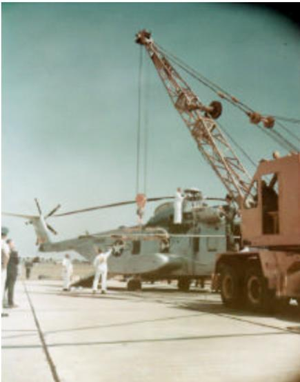
While crew 2 was removing the tail rotor blades and boxing them, mount bolts and rotor-head sling went into the blade shipping box for safe shipment. The first crew's blade bolt remover/installer connected the rotor head sling to the crane as it was jacked up.
