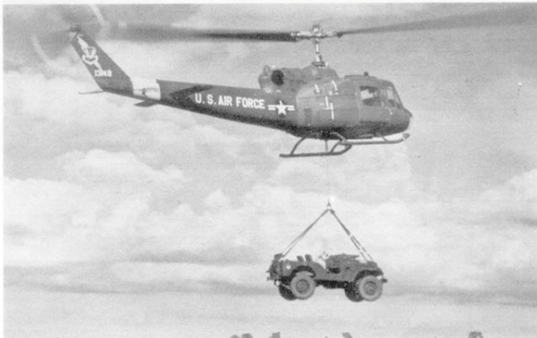
UH-1F of 4485th Test Wing lifts 2750 lb. jeep. T58-powered Bell helicopter weighs 4750 lbs. can lift loads as heavy as 4000 lbs.
